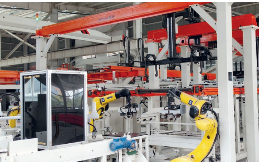
Automatic networking workstation
