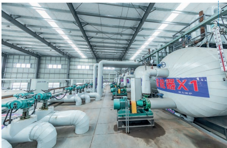
Residual steam recovery system.
