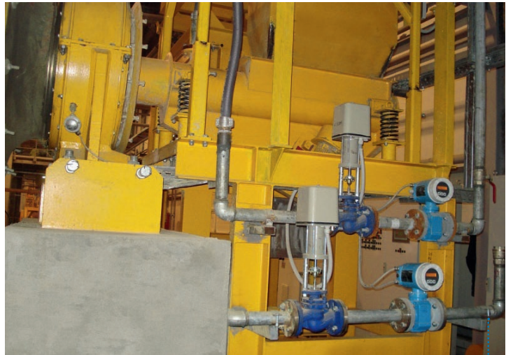
Precise control of the proportion of fresh water and condensate by means of two separate dosing units (flow measurement and regulating valve).
