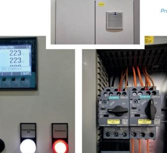
Properly marked: Warning lights and uniform labelling lead the plant operator to the cause of failure directly.
