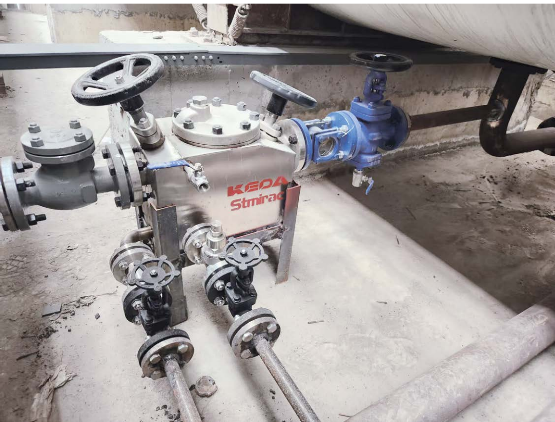
The Keda EcoSteam drainage system features a purely mechanical structure.
