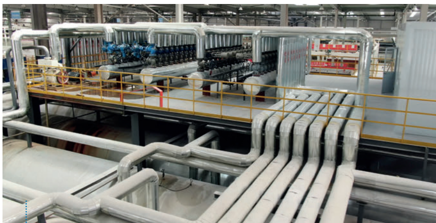
The BBMG Shanxi project has implemented an autoclave automatic control system to fully utilise steam and waste heat.
