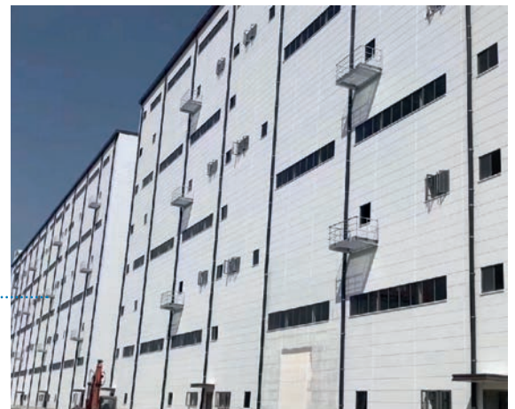
Fig. 1: AAC panel application in China.
