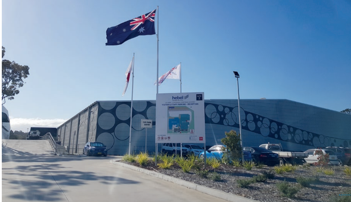
Fig. 2: The new facade of the second factory hall, utilizing routed 6-meter AAC wall panels
