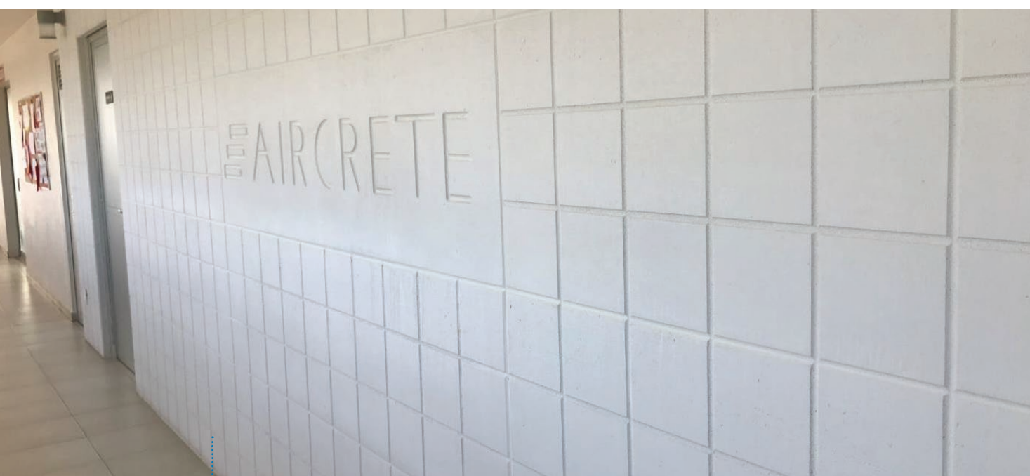
Fig. 9: Texts and even logos can be milled on AAC cladding panels with the Aircrete surface panel milling system.
