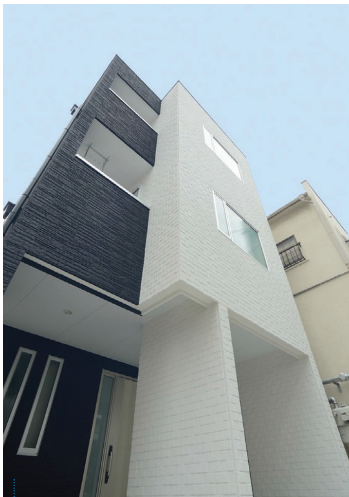
Fig. 1: The superior earthquake-resistance performance, insulation qualities as well as its ease of installation have made AAC cladding panels a first choice for many residential construction projects in Japan [2].
