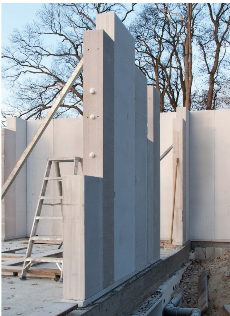
Fig. 1: The diverse prefab AAC elements of the Aircrete Building System incorporate usage of different sized panels, in line with the building drawings and plans.
