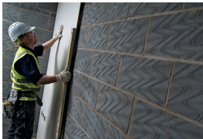
Fig. 2: Most AAC products in the UK are made using fly ash, giving the product its grey colour
