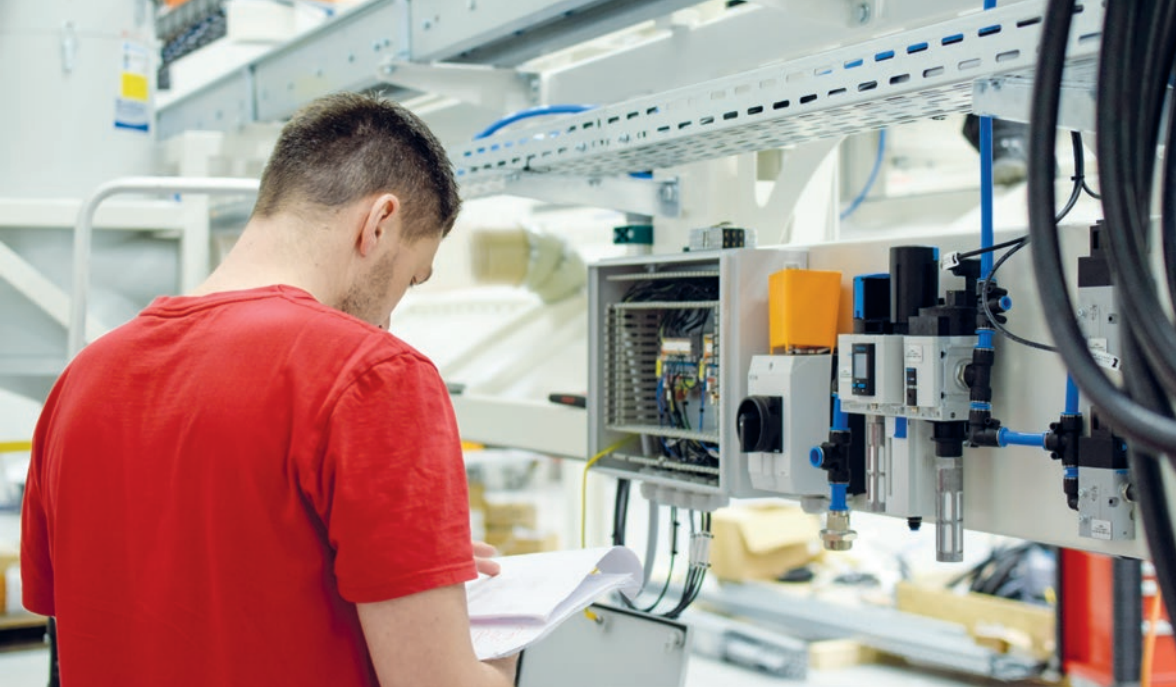
Fig. 5: Inspection of electrical and pneumatic control system during commissioning.
