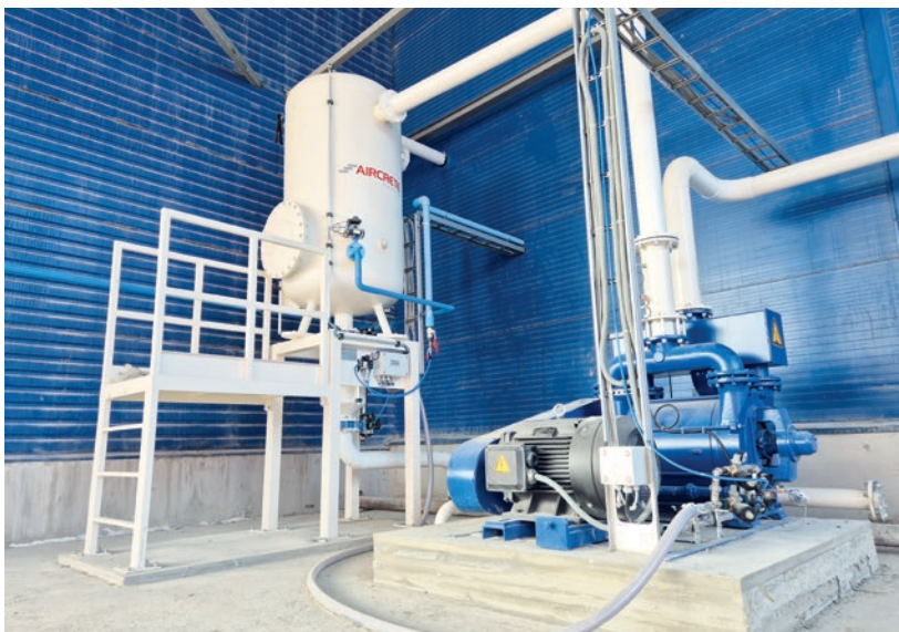
Fig. 1: Complete vacuum system installed at Bauroc's AAC plant in Matuizos, Lithuania.
