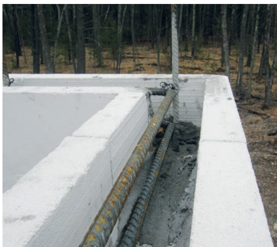
Ring beam including reinforcement
