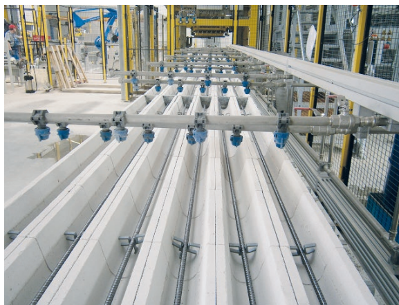
Irrigation station moistening U-blocks before concrete pouring to improve bonding and filling quality
