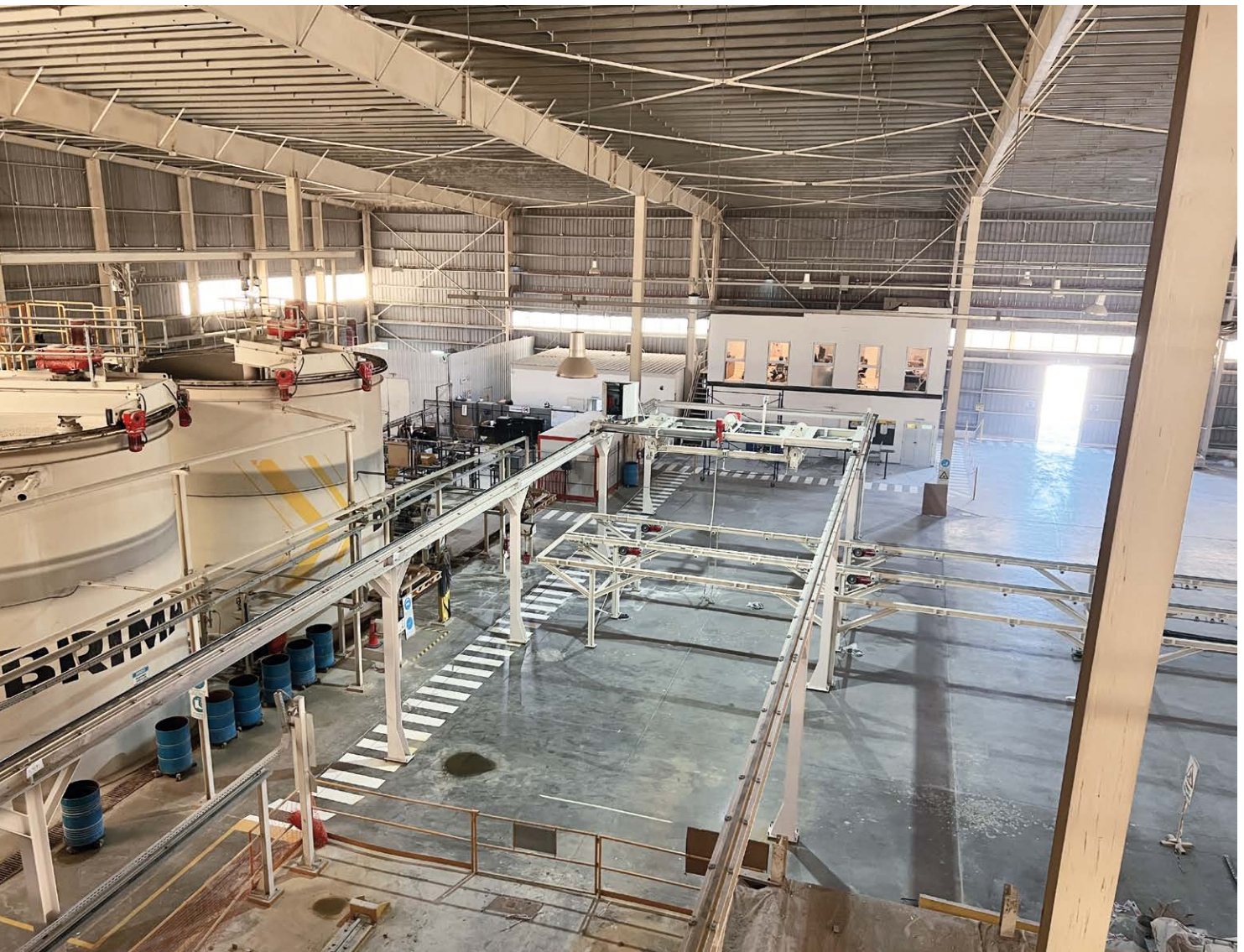
Fig. 4: Installed reinforcement manipulators gantry with the reinforcement manipulator at an end position in the far back.
