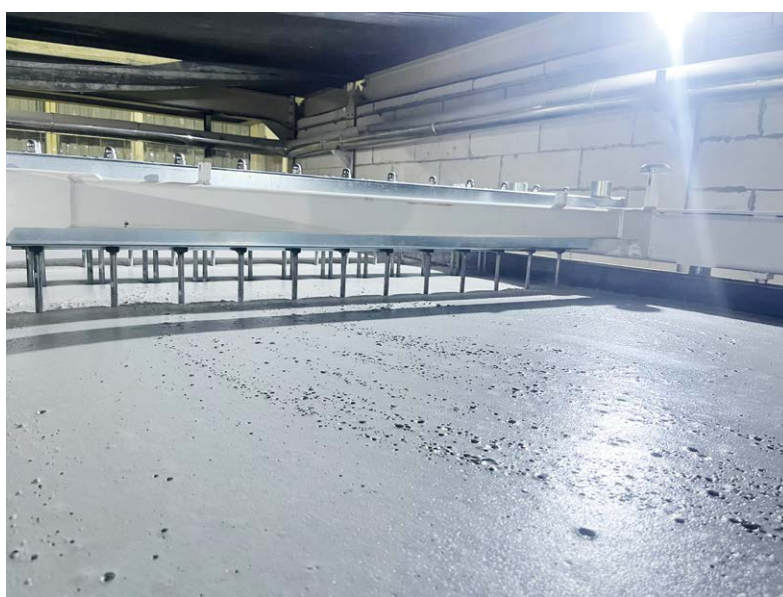
Fig. 6: Moulds with inserted reinforcement holding frames in the rising area.
