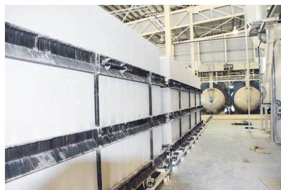
Fig. 9: Hardened cakes stacked 3-high after autoclaving.
