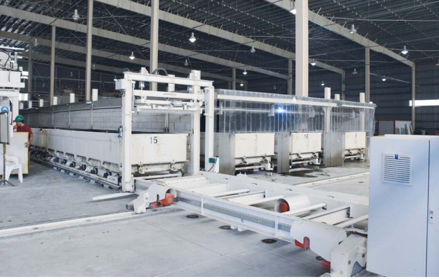
Fig. 3: View of the covered rising area.
