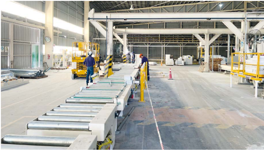
Fig. 10: Installing the additional line of conveyors for panels unloading.
