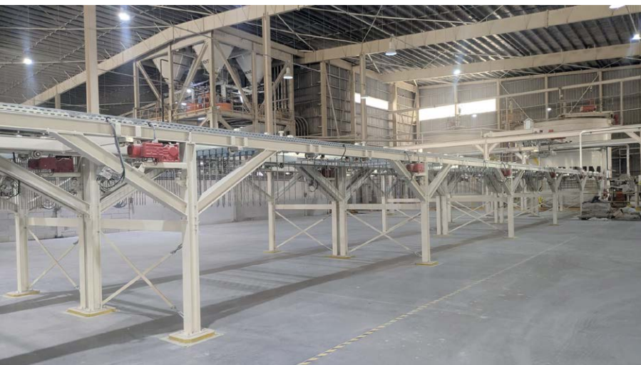
Fig. 5: Reinforcement holding frames with needles, waiting for cleaning on the reinforcement buffer line.
