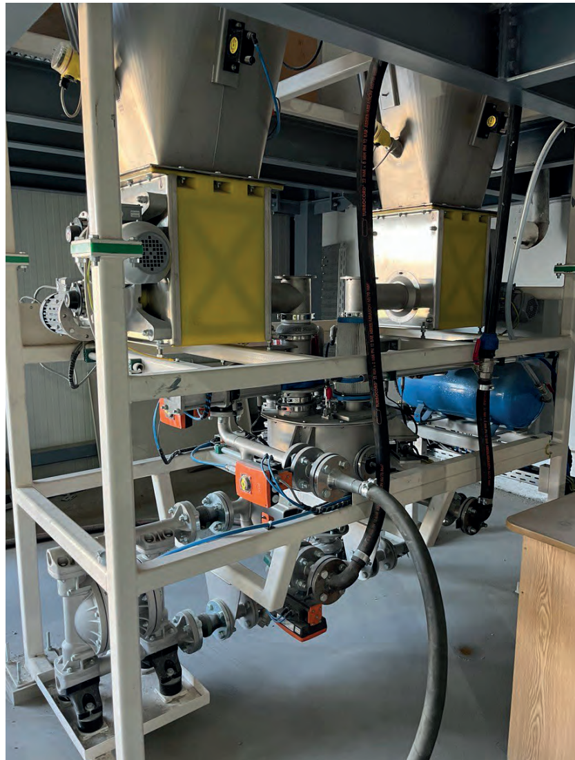
Fig. 4: New aluminium paste dosing system at Holcim, Romania
