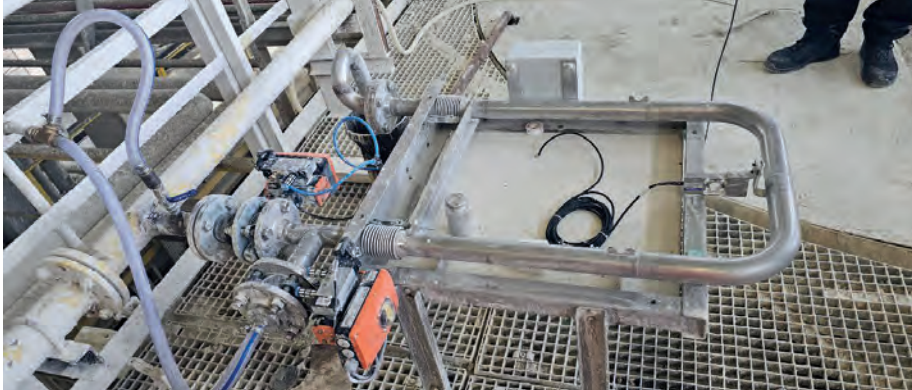
Fig. 3: New generation slurry density measuring system at an Aircrete customer in Türkiye
