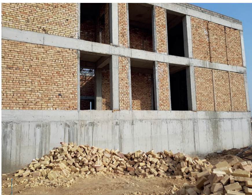
Fig. 8: Current way of building with red clay bricks is very labour intensive, leaves a lot of waste and requires extra reinforcement
