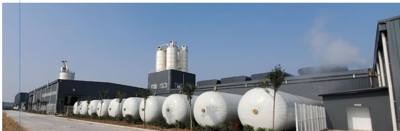
Fig. 3 and 4: The new plant of Luoyang Evergreen Building Technology is designed for a yearly capacity of 500,000 m 3 with 10 autoclaves
