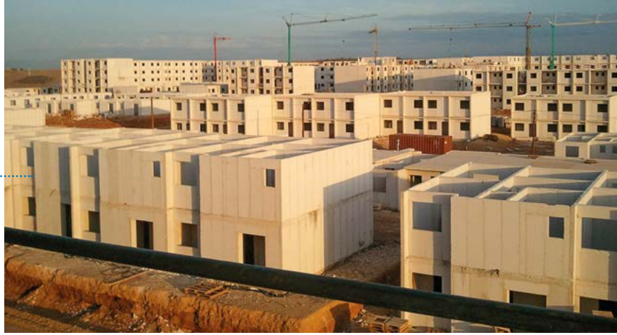
Fig. 2: The large housing projects in Sumbe, Angola are realized with AAC panels to create a modular, efficient and affordable building solution by Kora Angola [6].
